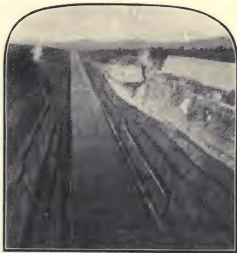
FIG. 246 The Ship Canal, Corinth, Greece
